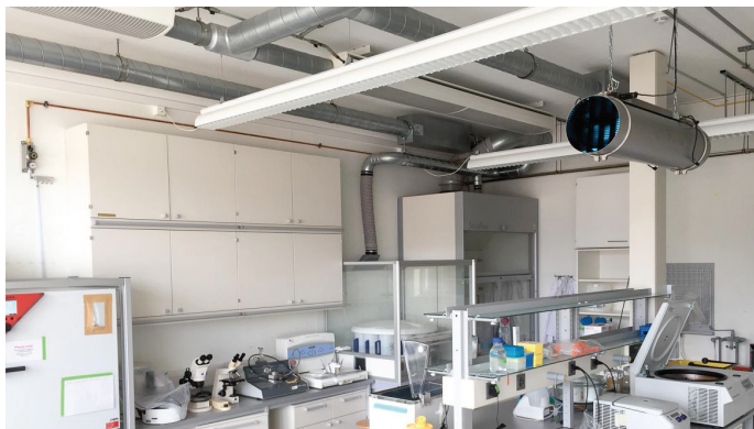
Laboratory with air recirculation system UVR-4K Air disinfection up to 700 m³/h
